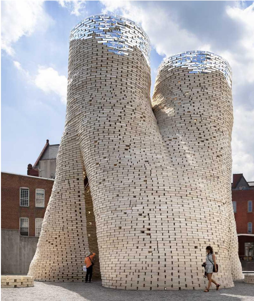
FIGURE 8: 15th edition of YAP (Young Architects Program), Hy-Fi . The temporary structure will be built using 3M reflective bio-design organic bricks, made from corn stalks and living root structures. The bricks will be used as growing trays before being used in the structure. Long Island City, 2014.
